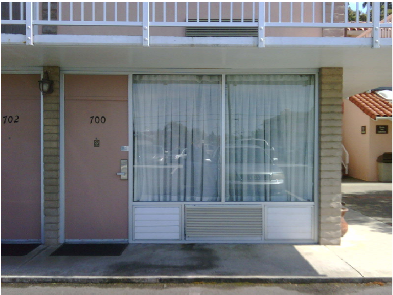
Figure 1. Photograph of the hotel façade discussed in the case study.
