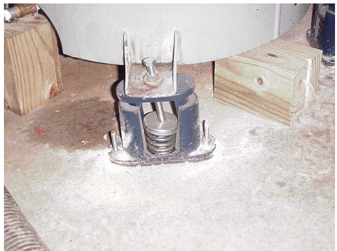
Figure 4: Springs supporting mechanical equipment collapsing, and with isolation efficiency reduced due to binding at side-bar restraints
