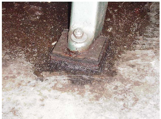
Figure 5: Mechanical equipment isolation (neoprene pad) efficiency reduced due to through-bolting
