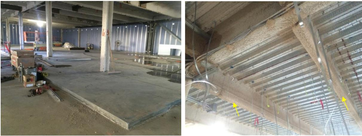
Figure 5: Case 3 – Photos of topping slab (left) and tube steel stiffeners from below (right, with fireproofing applied)
