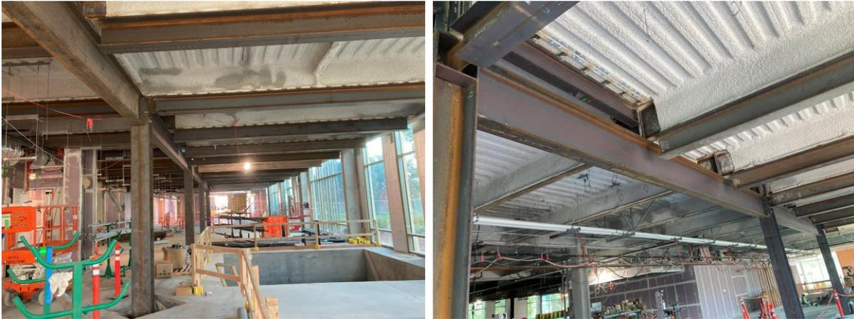
Figure 7: Case 4 – Stiffening steel and new columns and girders.
