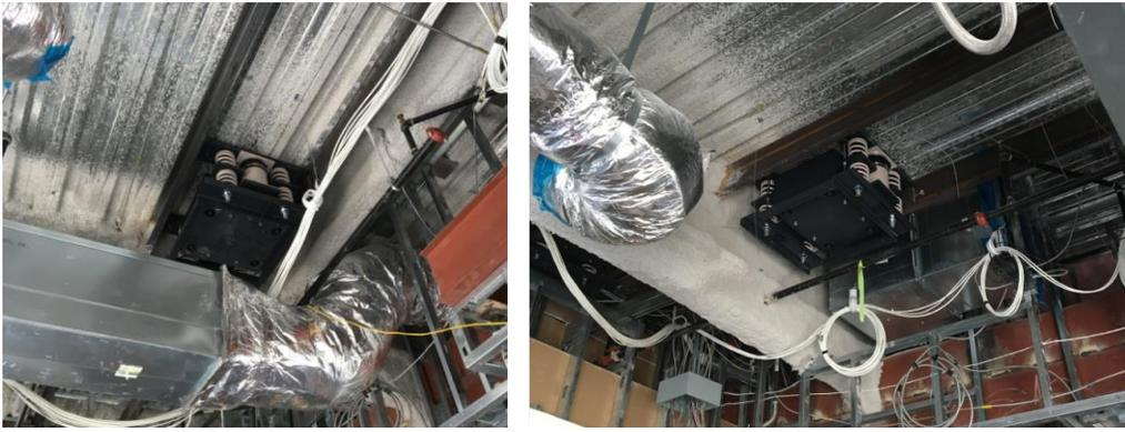
Figure 14: Case 6 – Tuned mass dampers mounted to the underside of the floor structure.
